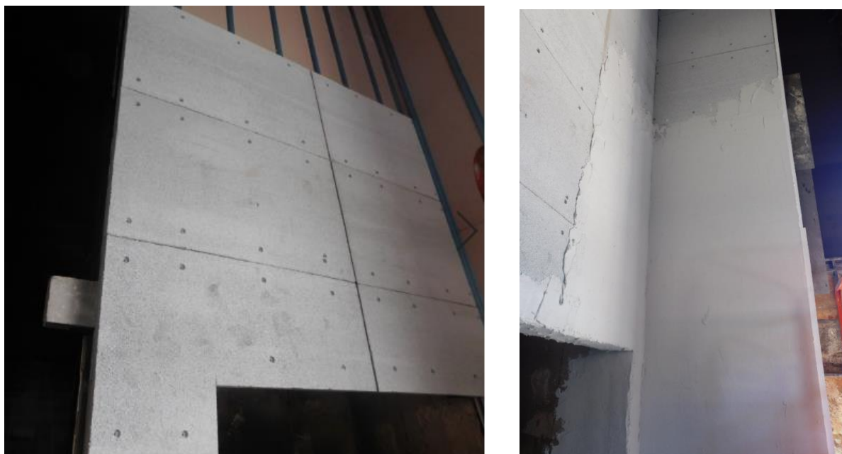
QT AND U-STUCCO™ FRX SYSTEM INSTALLATION
